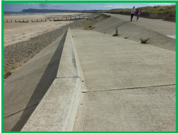
Slipway in very good condition at The Stray (/C0603C01).
