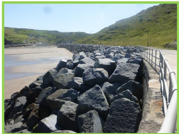
Modified rock revetment protecting inner face of jetty (Asset Ref No. 1221D901D0202C01)
