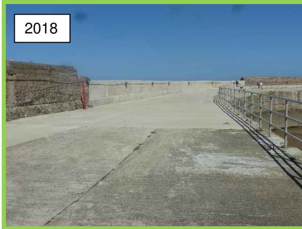
Repaired and improved structure in 2018 (Asset Ref No. 1221D901D0201C02)
