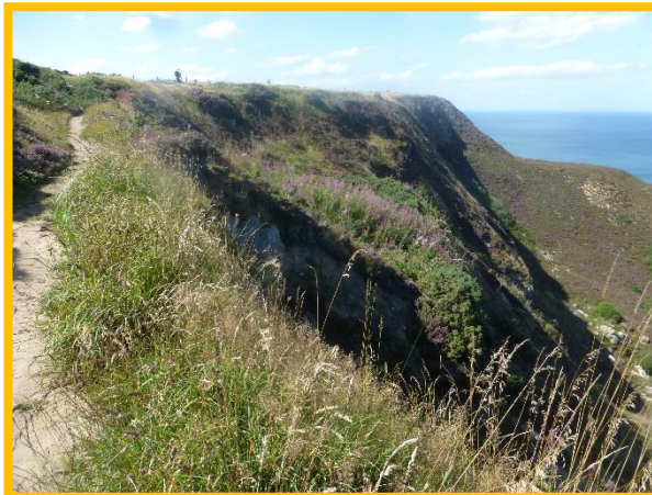
E58/2 Upper showing signs of ongoing headscarp recession.
