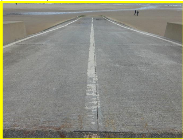
Slipway in fair condition (/C0602C02)
