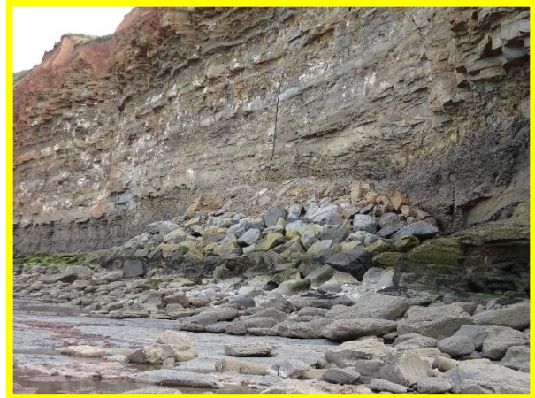
E60/1b Rock armour located at toe of cliff to the north of Cowbar Cottages
