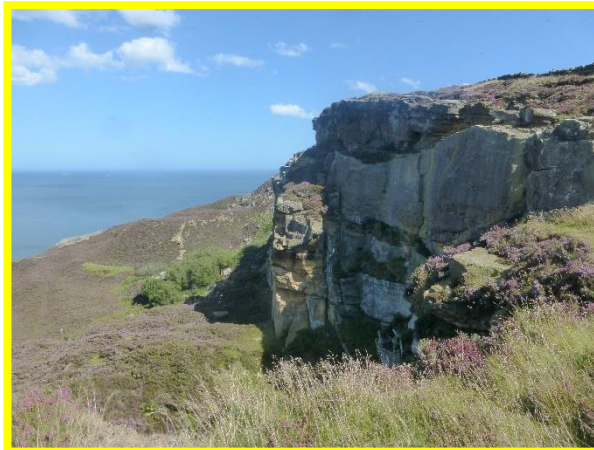
E58/5 Upper looking towards Rock Cliff. Locally Active upper sections and Partly Active lower sections.
