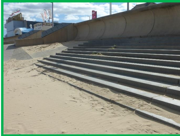
Stepped concrete revetment and recurve wall in very good condition (/C0602C03)
