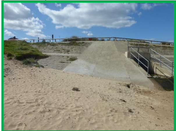
Transition of revetment into natural defence (/C0603C01)
