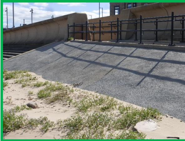
Slipway on in very good condition (/C0602C04)
