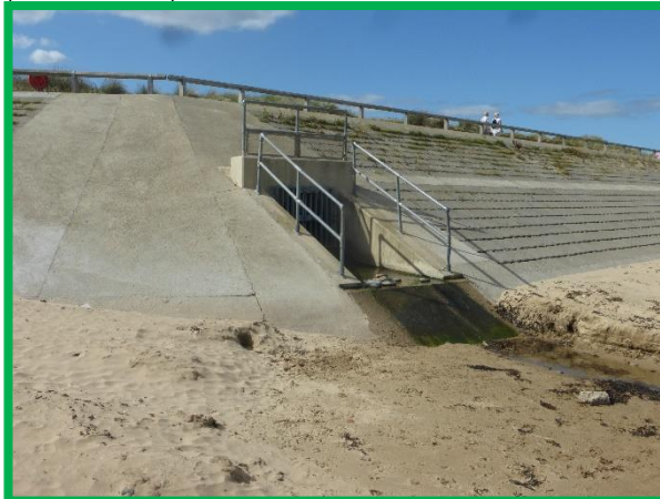
Outfall at south eastern end of (/C0603C01)
