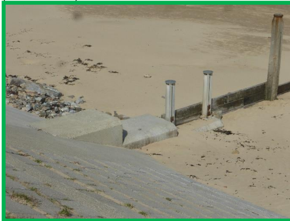
Recently repaired groyne along The Stray (/C0603C01)
