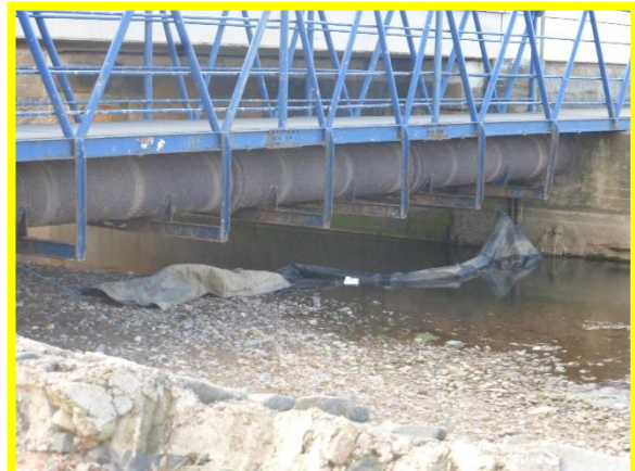
Silt curtain installed at Skelton Beck.
