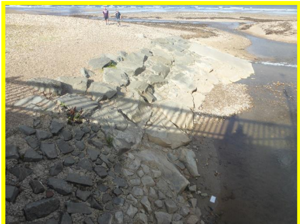
Grouted rock revetment in fair condition (/C0704C06)
