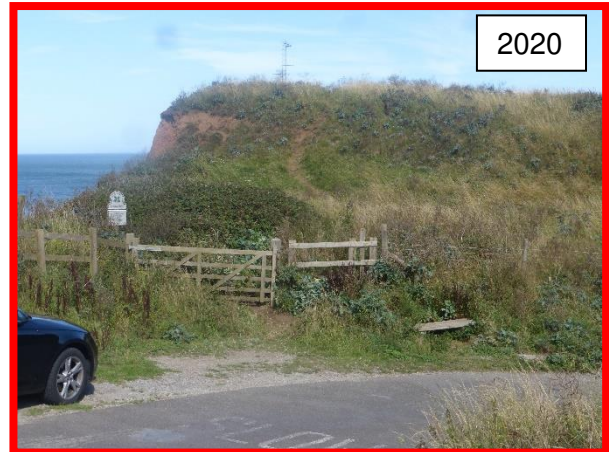
E60/1 In 2020 the access is now no longer marked as closed although the path onto the Nab is overgrown.
