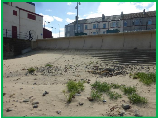
Accumulation of beach material at transition with cinema wall (/C0602C06) & (/C0602C05)
