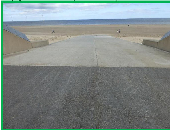
Slipway in good very condition (/C0602C03)
