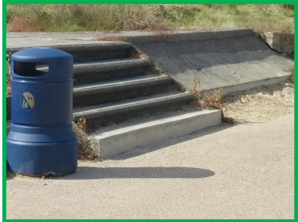
Recently repaired step at The Stray (/C0603C01)
