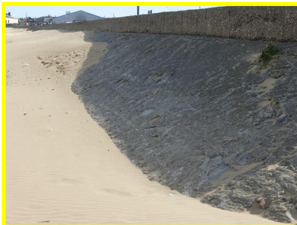
Grouted stone revetment, partially covered due to high beach levels (/C0601C01)
