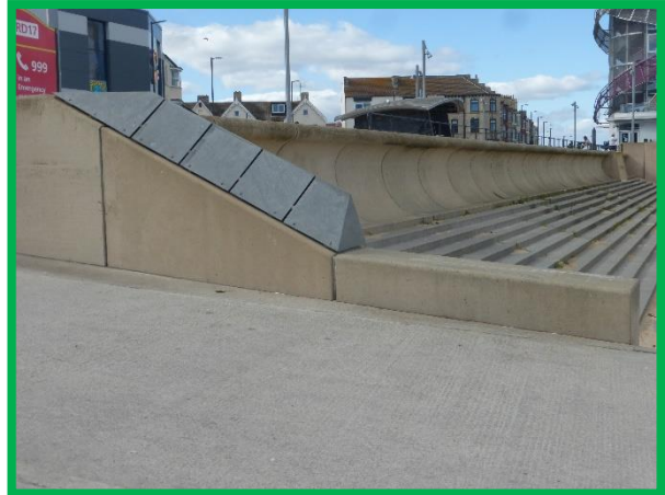
Stepped concrete revetment and recurve wall in very good condition (/C0602C03)
