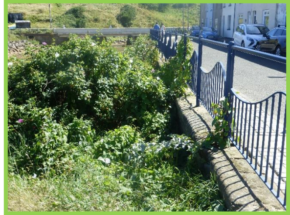
Blockwork wall at rear of revetment (Asset Ref No. 1221D901D0202C02)
