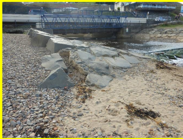
Exposed crest of grouted rock revetment (/C0704C06)
