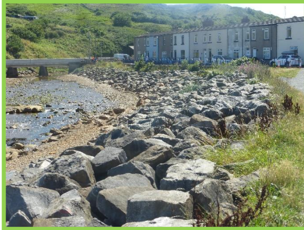
Rock armour revetment fronting properties . (Asset Ref No. 1221D901D0202C02)
