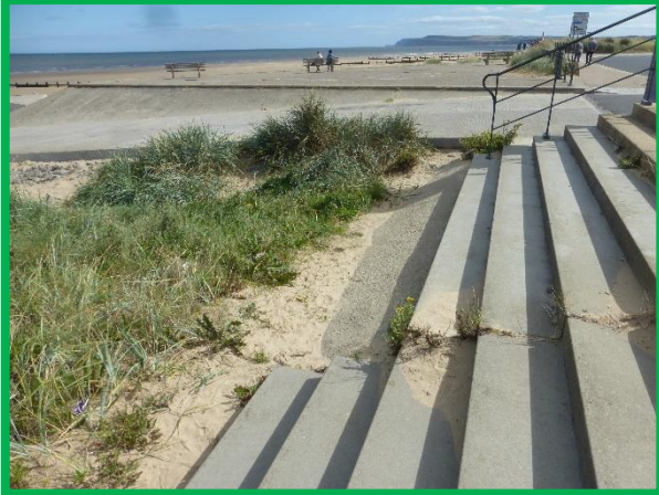
Vegetation growth indicating long term accretion at the slipway (/C0602C01)
