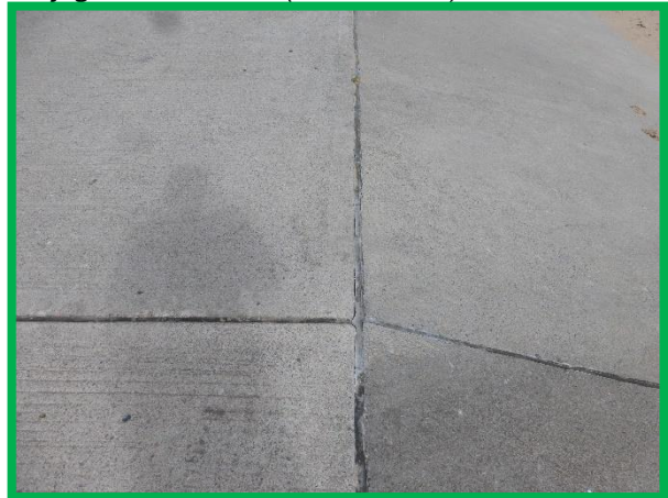
Joint sealant on slipway remains in good condition (/C0602C03)
