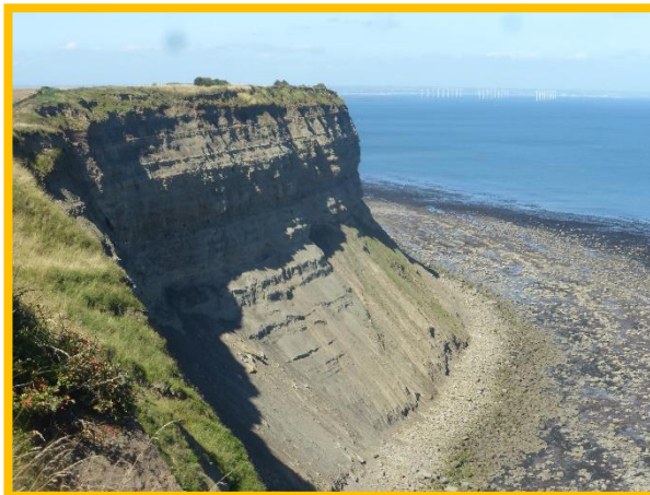
E54/4 looking northwest along Hunt Cliff showing active cliff face and debris apron (Partly Active)
