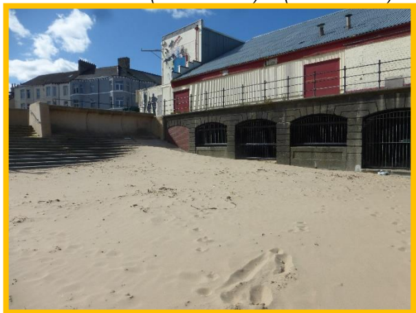
Cinema seawall note accumulation of beach material (/C0602C05)
