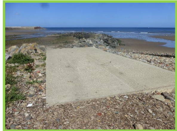
Rock armour groyne and concrete slipway (Asset Ref No. 1221D901D0202C05)
