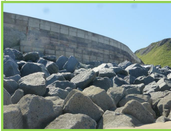
Seaward face of repair. (Asset Ref No. 1221D901D0201C02)
