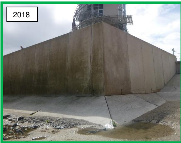
Concrete sea wall at Redcar Beacon in 2018 (/C0602C03)
