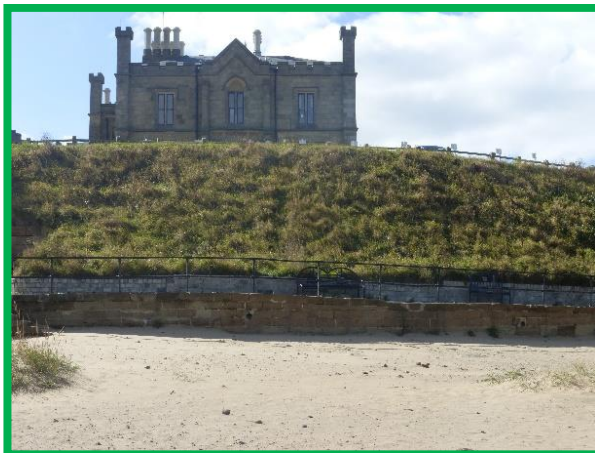
Vegetated slope above masonry wall CBU E52/7
