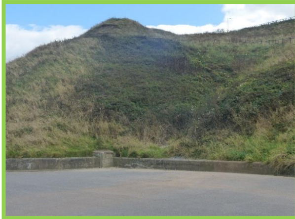
View looking east (E52/3b)
