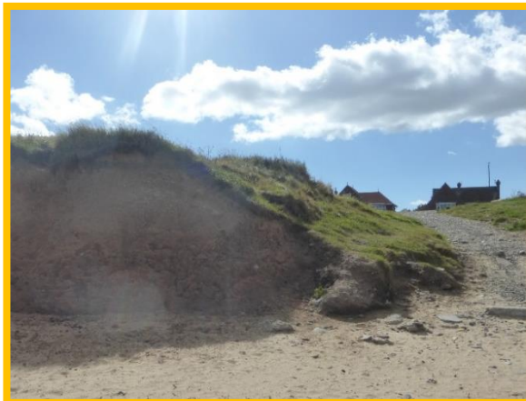
CBU E52/10 (left) and informal access ramp (right)
