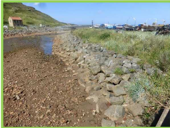
Rock armour protection along eastern edge of Kilton Beck. (Asset Ref No. 1221D901D0202C05)
