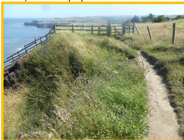
E58/1a headscarp recession encroaching on footpath.
