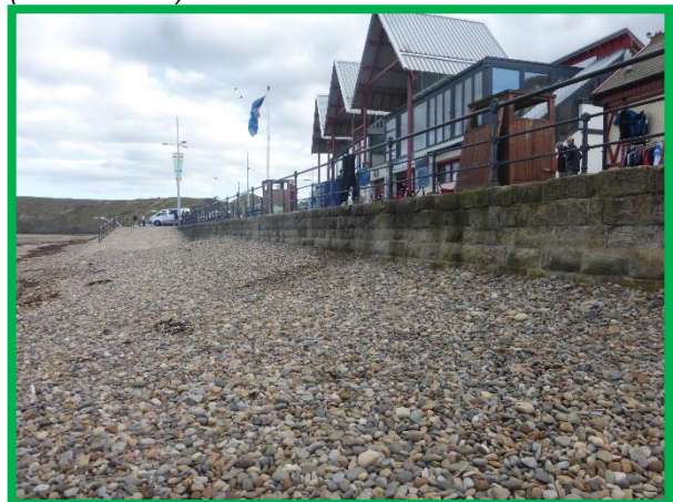
Looking south east along masonry wall south of pier (/C0702C04).
