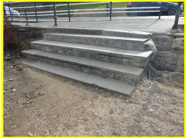
Repairs to steps in fair condition (/C0704C06)
