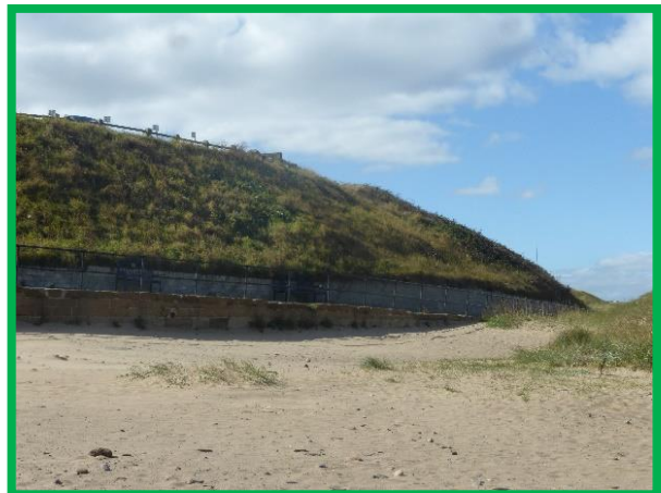
Vegetated slope above masonry wall CBU E52/7
