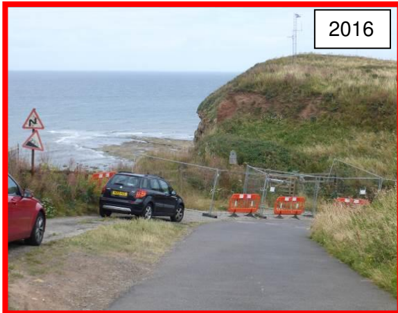
E60/1 Closure of access to Cowbar Nab in 2016, in 2018 the access appeared in very similar state with the same Heras fencing and plastic barriers still in use.
