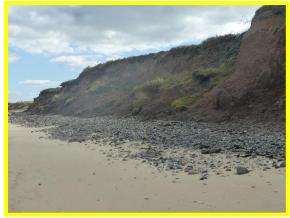
View looking south east CBU E52/9
