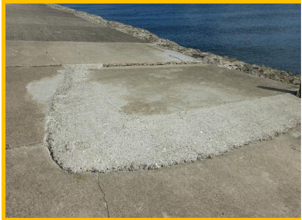
Recent repair to deck slab along eastern face (/C0506C01)
