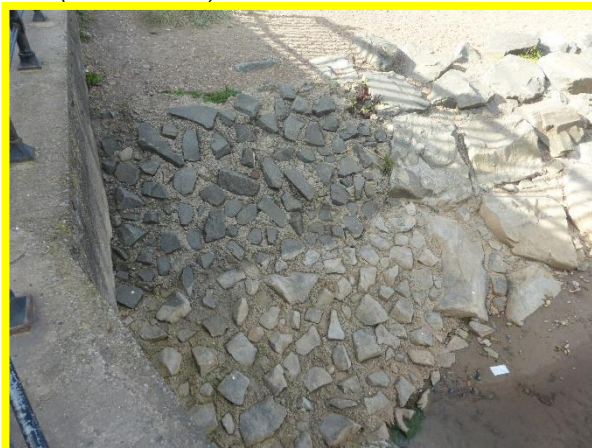
Grouted rock revetment in fair condition (/C0704C06)
