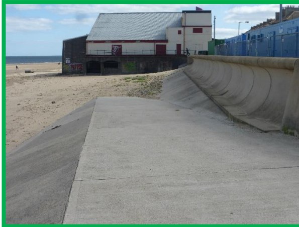
Slipway in good condition (/C0602C06).
