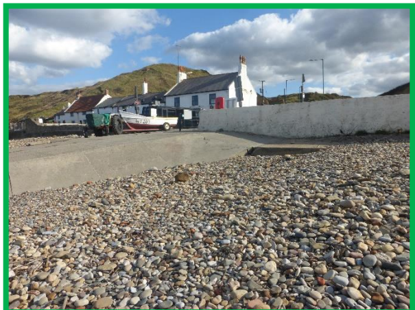
Western face of concrete slipway (/C0704C03)
