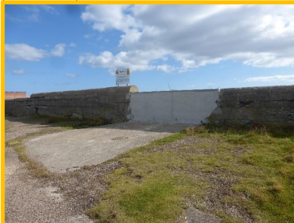
Repairs to wall on breakwater crest (/C0506C01)
